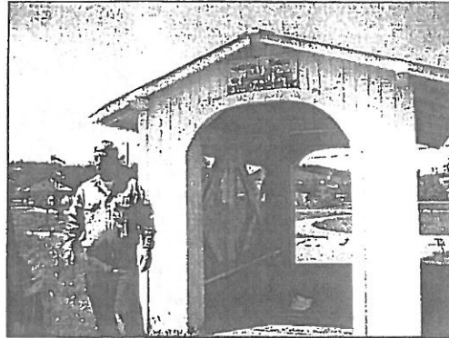
Mayor Warren Weathers in front of the Community Park's covered bridge
