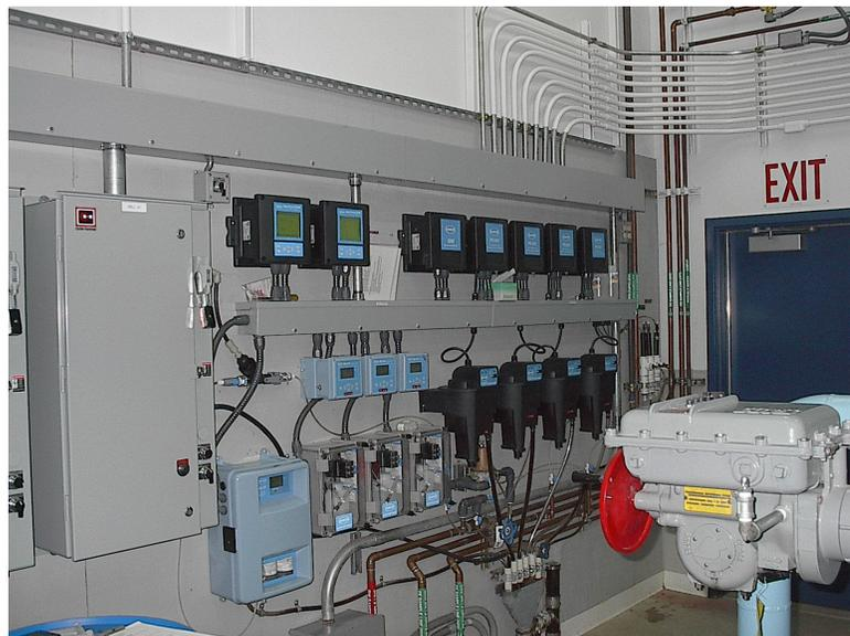
To correct this problem, the plant upgrade should consider relocating the instrumentation sensors closer to the sample points and/or using smaller diameter piping for the sample lines to increase the velocity in the sample piping.
