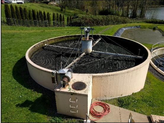
Trickling Filter at the Sewer Plant
